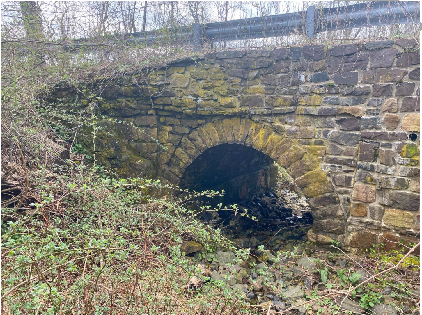
Photo 3: Northeast (upstream) side of the bridge, view facing south.
