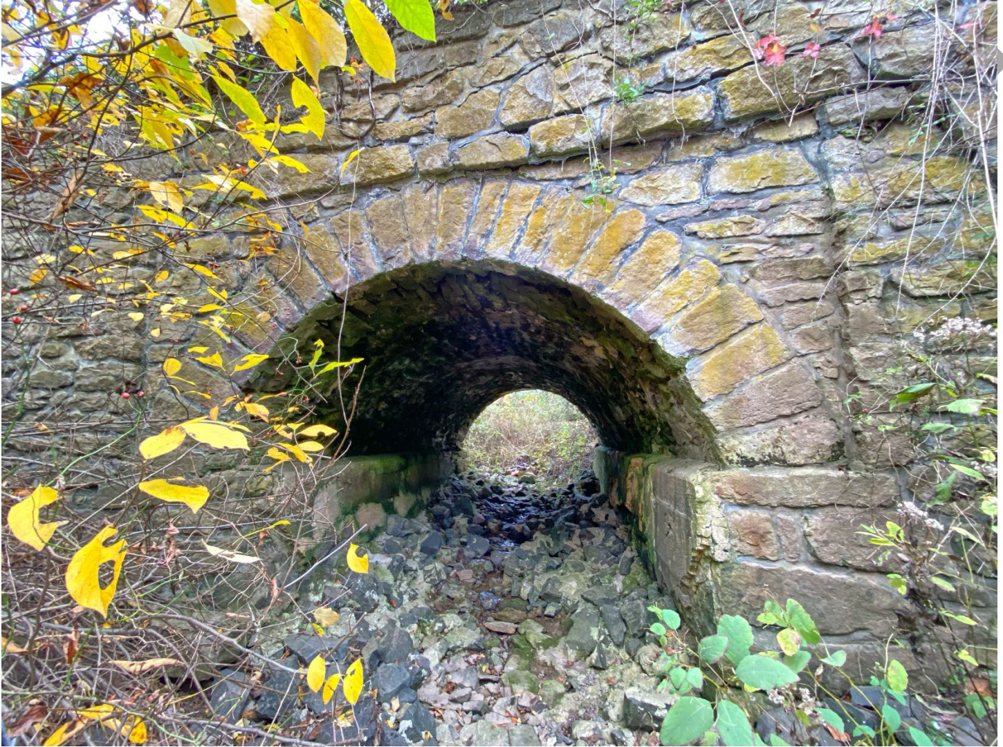
Photo 6: Southwest (downstream) side of the bridge, view facing northeast.
